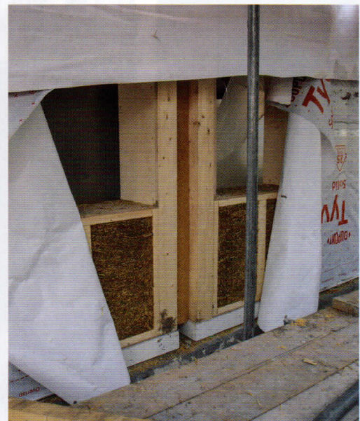
Prefab stropanelen achter folie.
